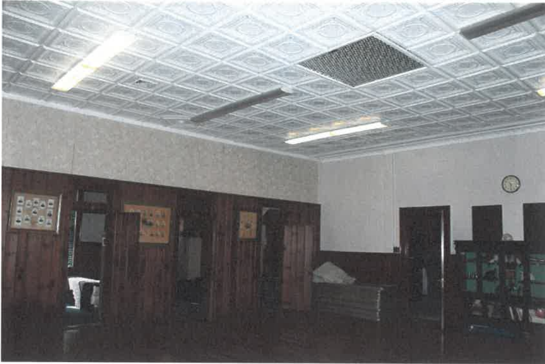
3.7 Second floor of fire station. Limited operational function
